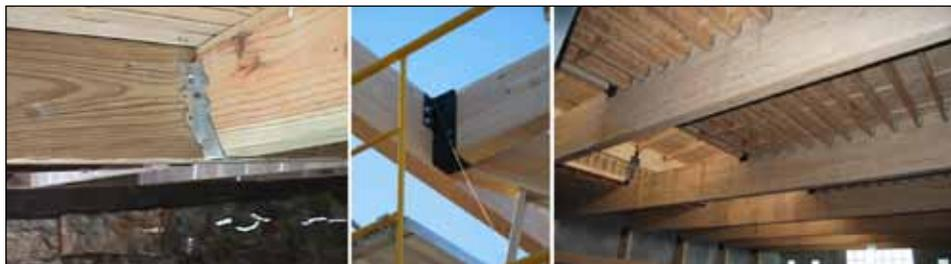
Figure 8-28. Typical joist hanger connectors.
